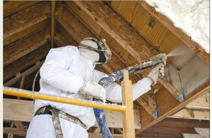
Application of SPF to the underside of sloped roof rafters
